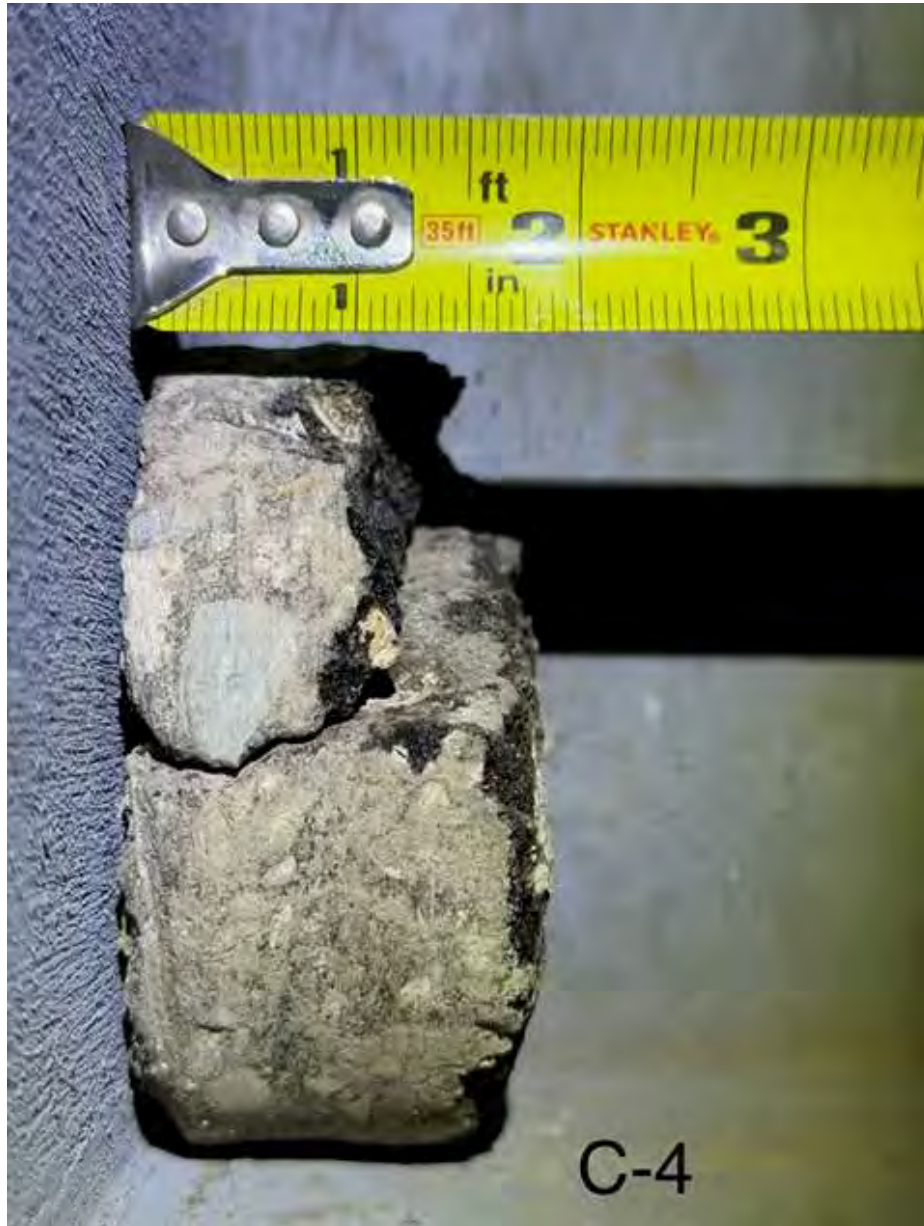
Photograph 4: Pavement Core C-4.
