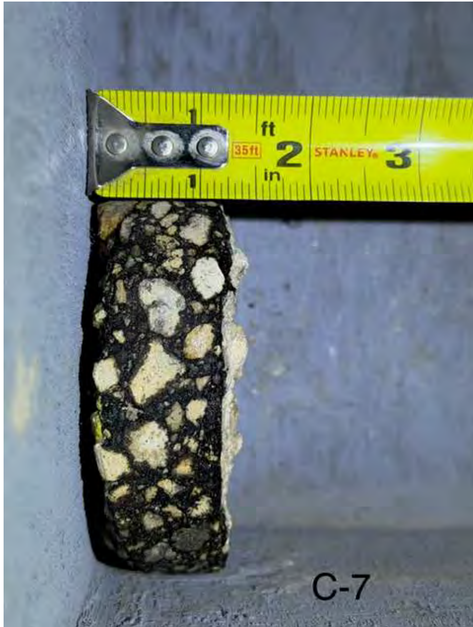
Photograph 7: Pavement Core C-7.
