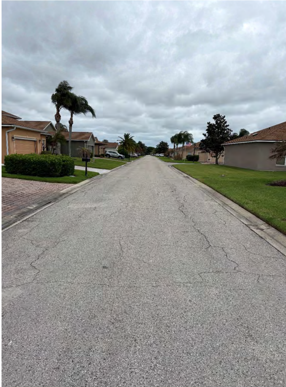
Photograph 9: Picture of pavement condition at the project site.
