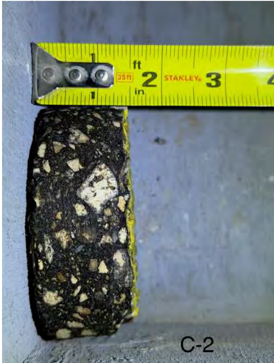
Photograph 2: Pavement Core C-2.
