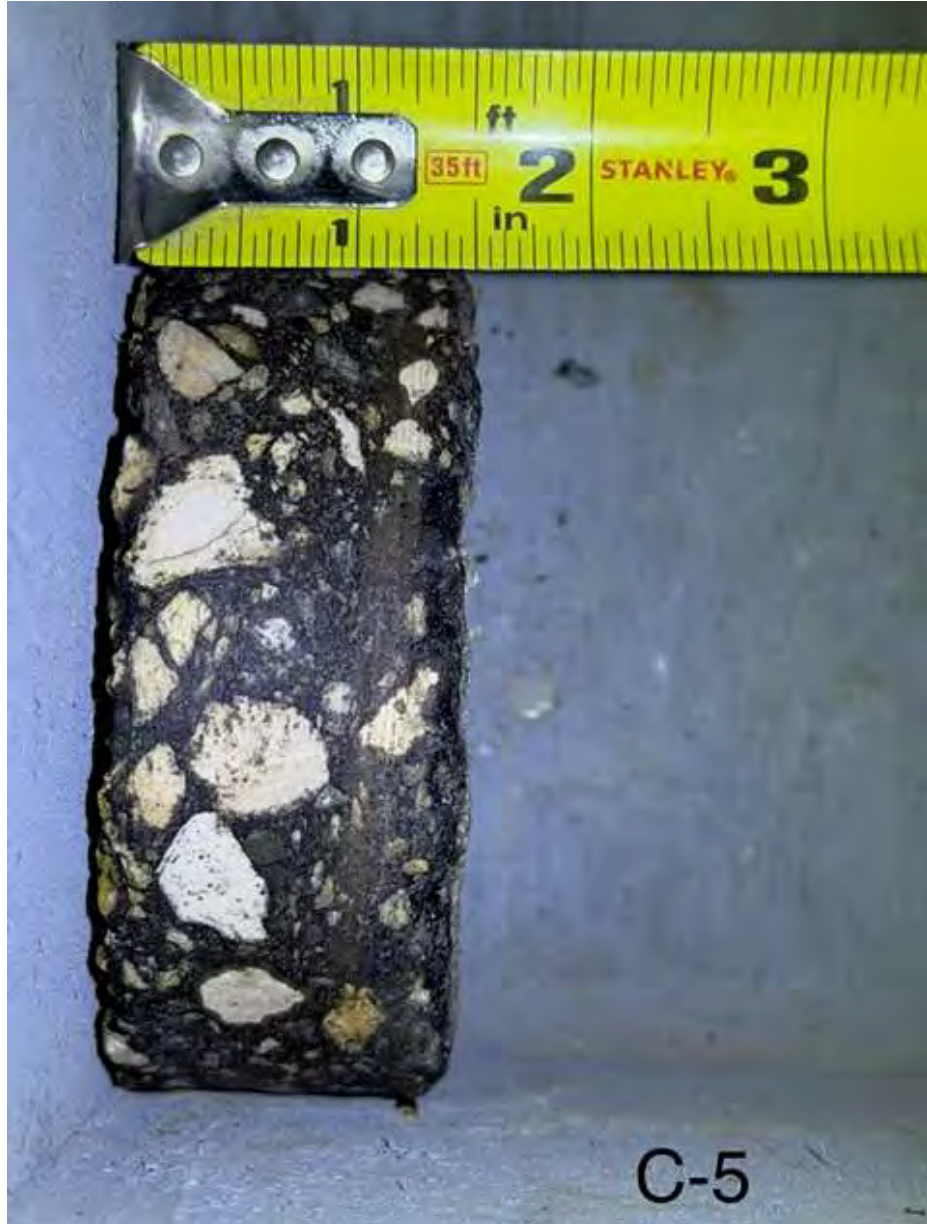
Photograph 5: Pavement Core C-5.
