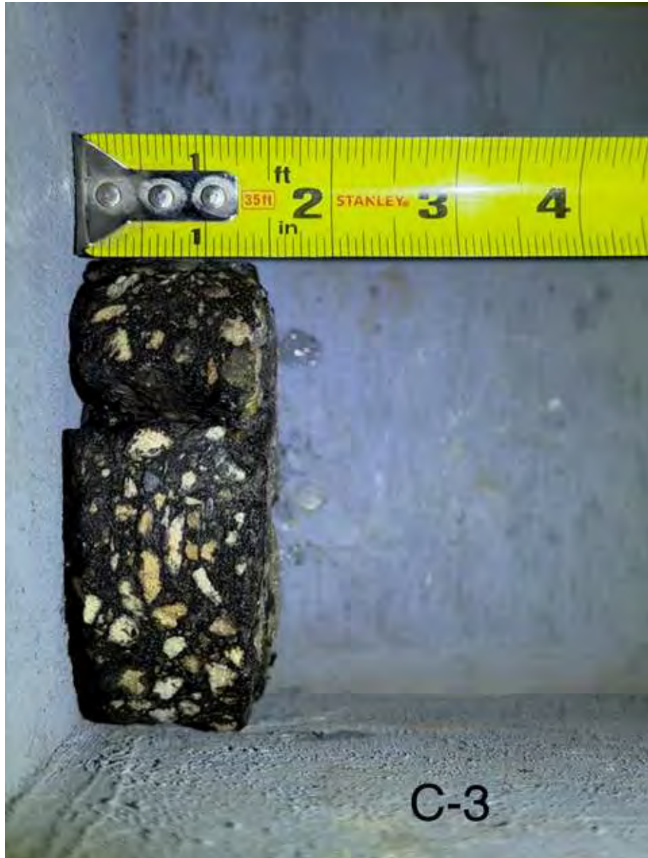
Photograph 3: Pavement Core C-3.
