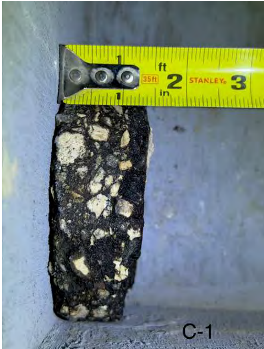
Photograph 1: Pavement Core C-1.
