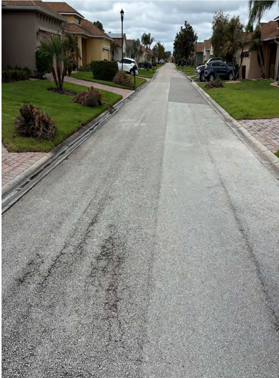
Photograph 8: Picture of pavement condition at the project site.
