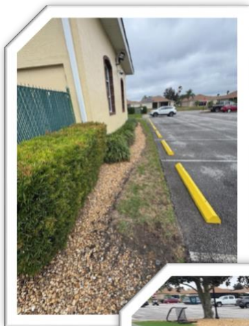
Sod being replaced in these location
