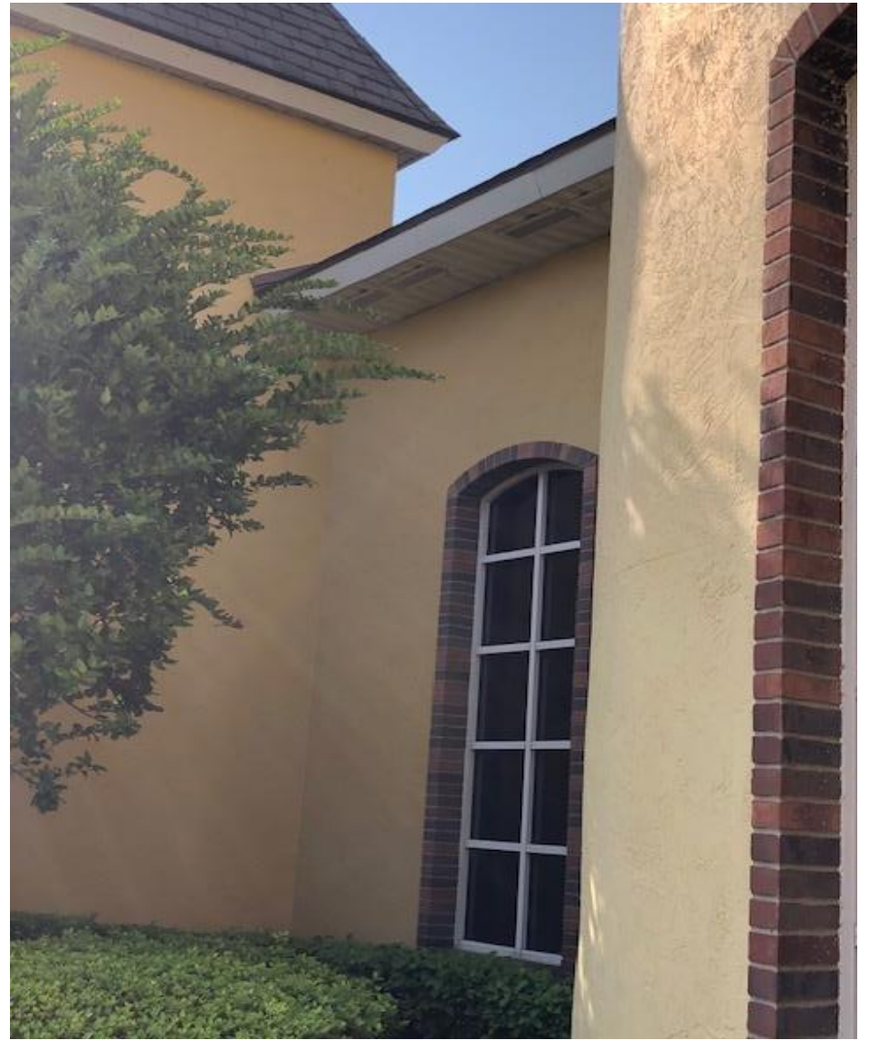
Additional area to install new gutter system
