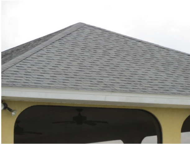
Pavilion asphalt shingle roof
