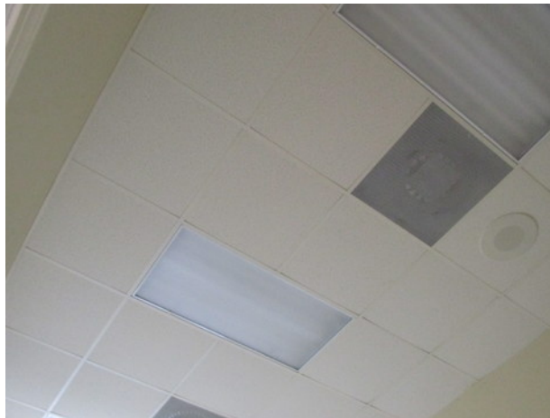
Typical acoustic ceiling tile and grid
