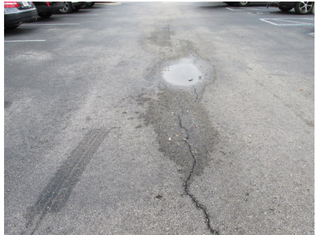
Clubhouse parking area with cracks and standing water
