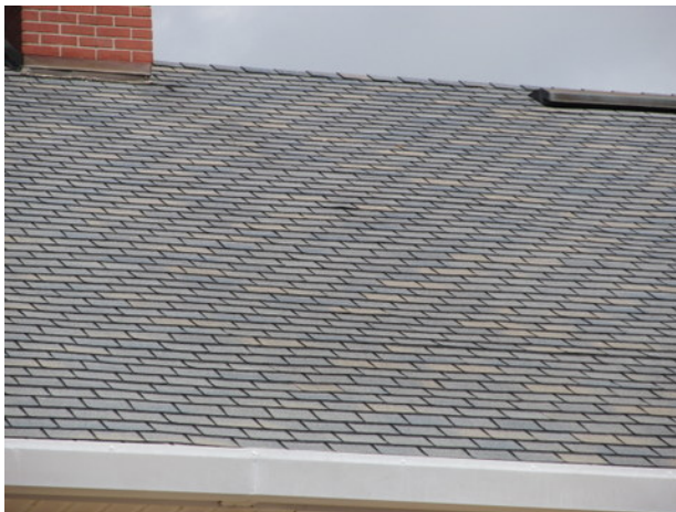
Clubhouse asphalt shingle roof with shingle lift
