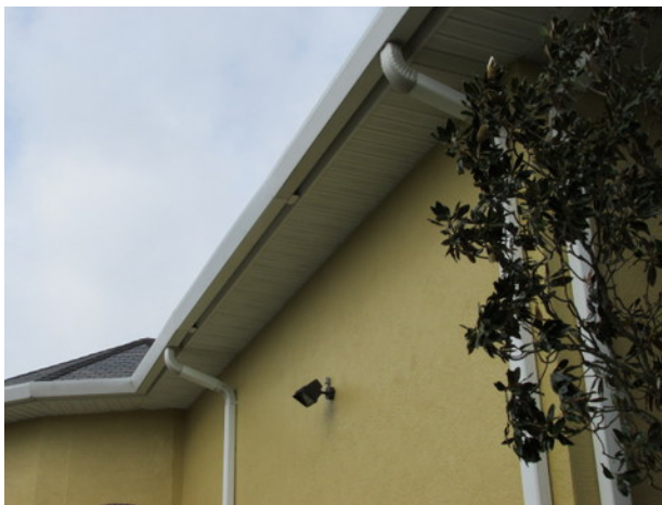
Typical gutter and downspouts
