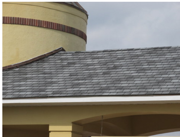
Guard house asphalt shingle roof
