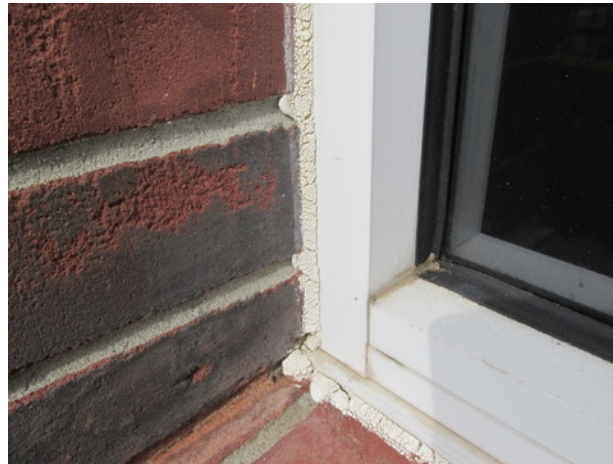
Clubhouse window with sealant deterioration
