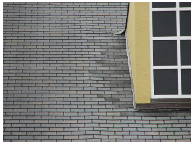
Clubhouse asphalt shingle roof with roof patch
