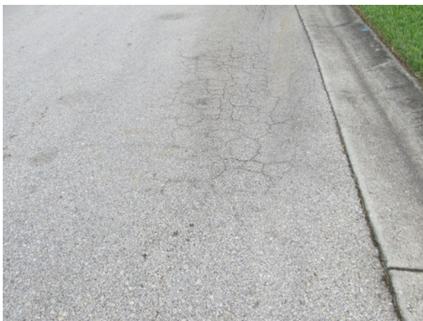
Asphalt pavement with alligator cracks
