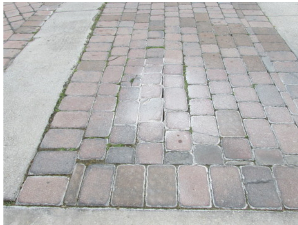
Cracked and settled pavers at Lake Ashton Boulevard
