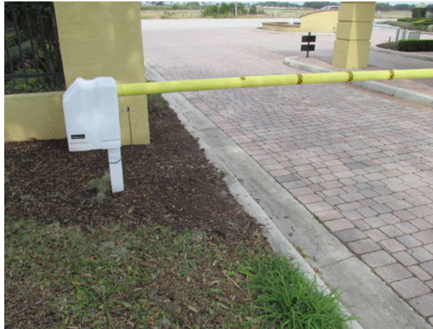
Typical gate arm and operator
