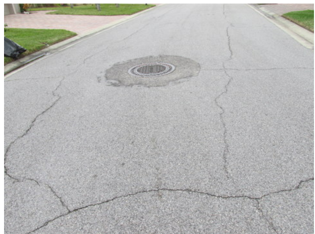
Asphalt pavement with block cracks
