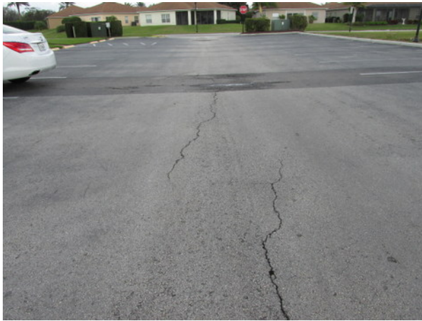
Clubhouse parking area with patch and cracks
