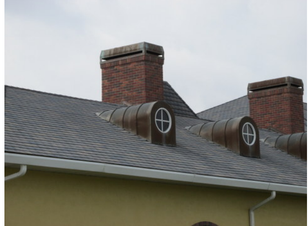
Clubhouse asphalt shingle roof
