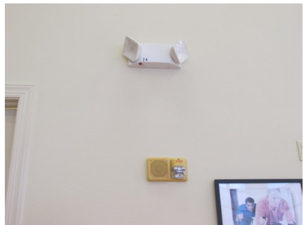
Typical life safety emergency devices
