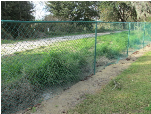
Typical chain link perimeter fence with leaning section
