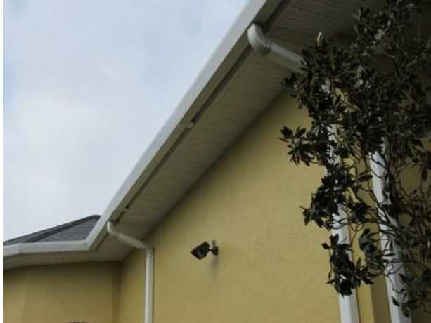
Typical gutter and downspouts
