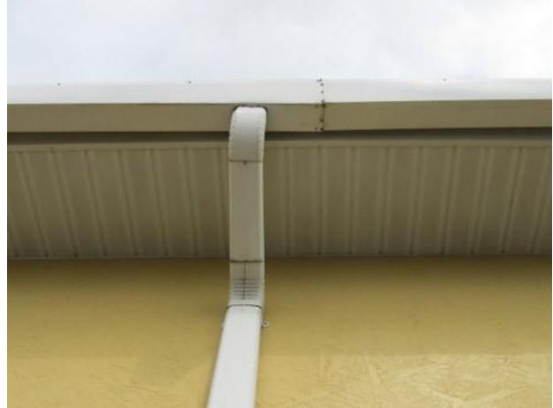
Gutter with dent
