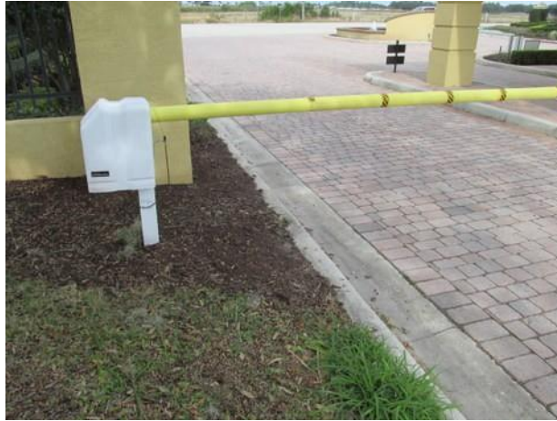
Typical gate arm and operator
