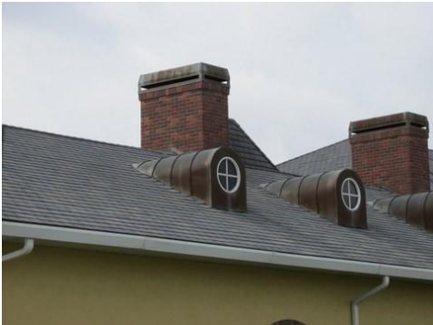
Clubhouse asphalt shingle roof
