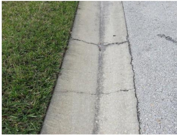
Gutter with cracks
