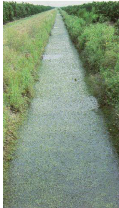
Figure 5. Southwest Florida citrus irrigation and drainage ditch with dense Hydrilla which blocks water movement.
