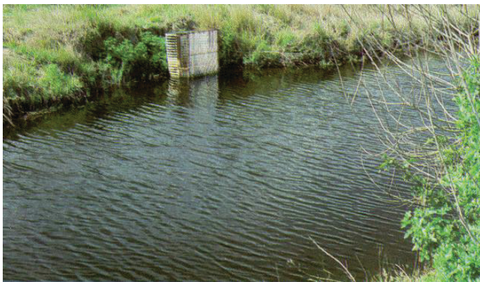
Figure 7. Fish barrier installed on a water control structure in a citrus irrigation and drainage canal. Fish barriers are used to manage unwanted grass carp movement in the agricultural waterways. Credits: David L. Sutton
